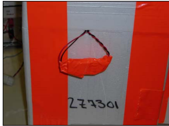
Figure 26 -Once connected wrap cables with tape
